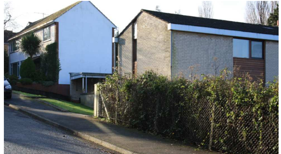
Plate 3. View from Bramble Drive towards no.5 which sits at the higher southern end of the application site.
